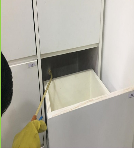
TERMITE TREATMENT IN PROGRESS
