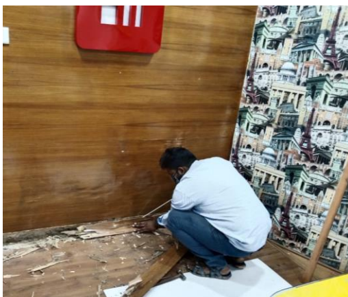
Repairs at GoGlobal
