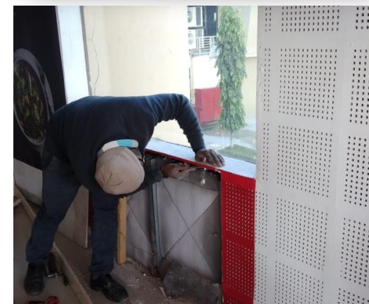
Repairs at Escoffier
