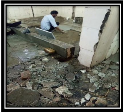
Kota stone fixing work at food court kitchen
