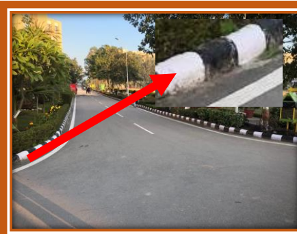
The curb stones had worn out and had patches Hence these were repaired by the Maintenance Team (Mason Work) April-May 2020. The work is in progress.
